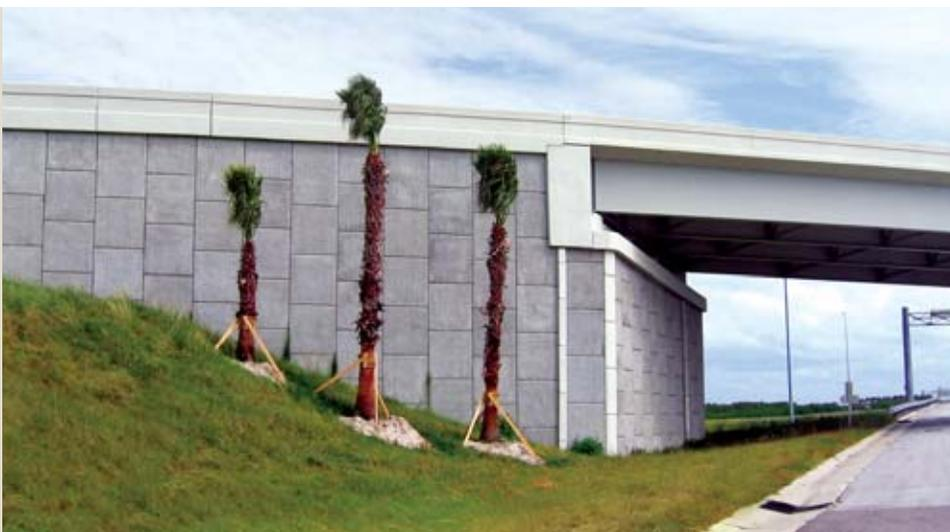
ARES Full-Height Panel Walls can be constructed over 30 ft. vertically with a single panel.
