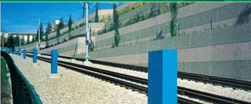
contractors have achieved sustained panel placement rates of up to 800 sq. ft. of wall per hour (site preparation and component staging are the keys to achieving these rates of construction). With good planning and proper coordination, one panel can be set every 12 to 18 minutes with an average of 32 panels in a two-hour shift.
